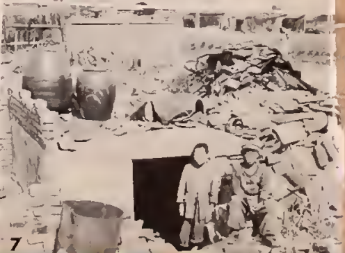
7. Seoul - 1951. Homeless waifs find shelter in a coal cellar.
